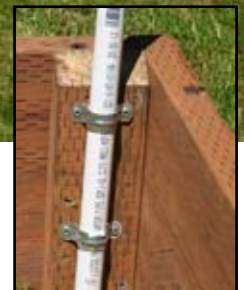
Figure 4 insert. Insert pipe straps.
