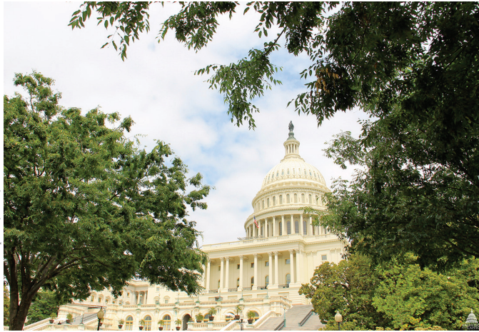
With well-designed state and federal policies and careful planning and coordination, the United States can greatly increase its clean energy resources, cost-effectively comply with the emissions reductions required by the Clean Power Plan, and reap important economic and public health benefits in the process.
